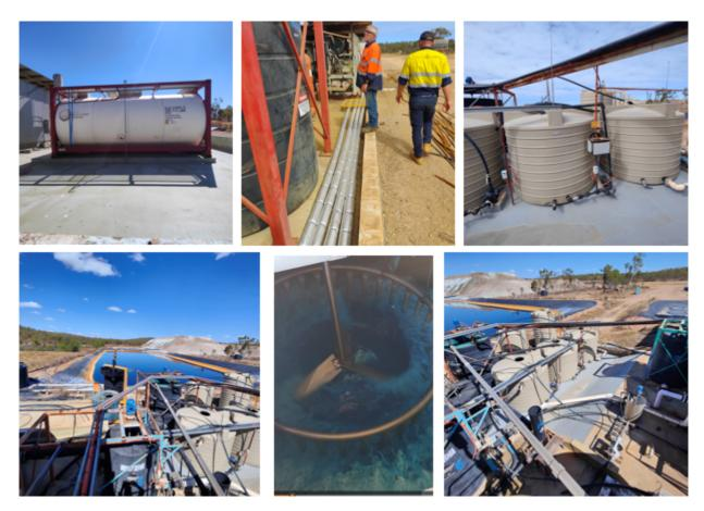
Figure 1. Tartana Solvent Extraction – Crystallisation Plant. Clockwise – New acid tanks with delivered acid, Inspection of pipework, New tanks for copper stripping, View of plant tanks and pipework, Copper sulphate crystals in crystalliser, Plant, PLS pond and heaps for leaching in distance.
